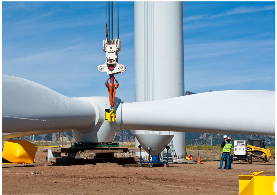
Drawing a wind turbine up for placement (Credit: Dennis Schroeder / NREL)
