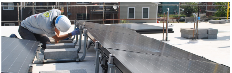
Working on a rooftop solar energy system Photo Credit. Jamie Nolan / U.S. Department of Energy
