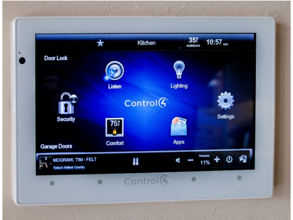
Home energy management system Photo Credit. U.S. Department of Energy
