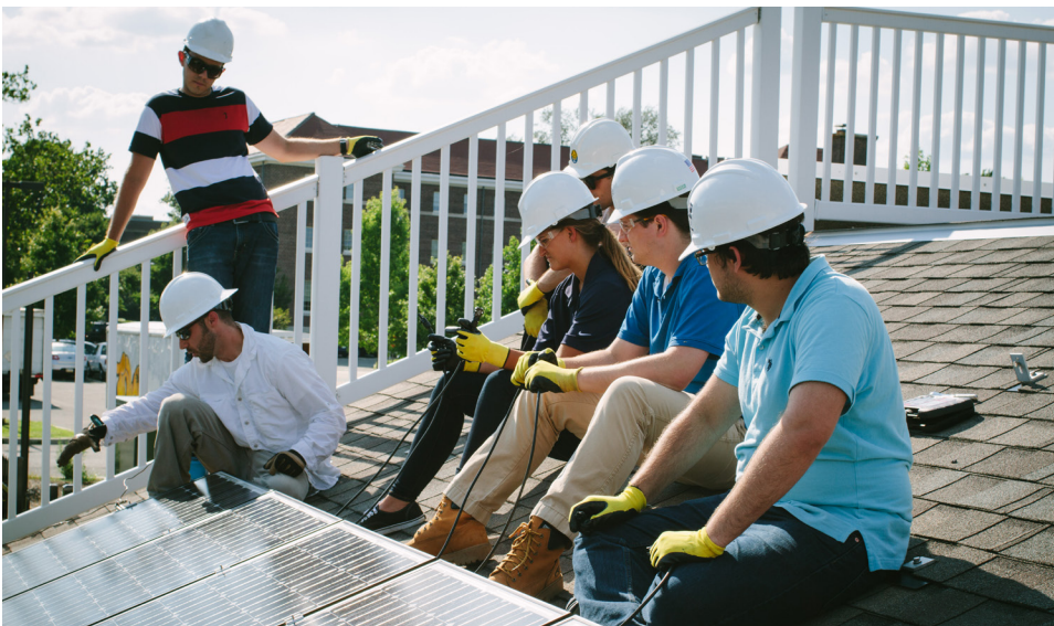
Solar rooftop training
