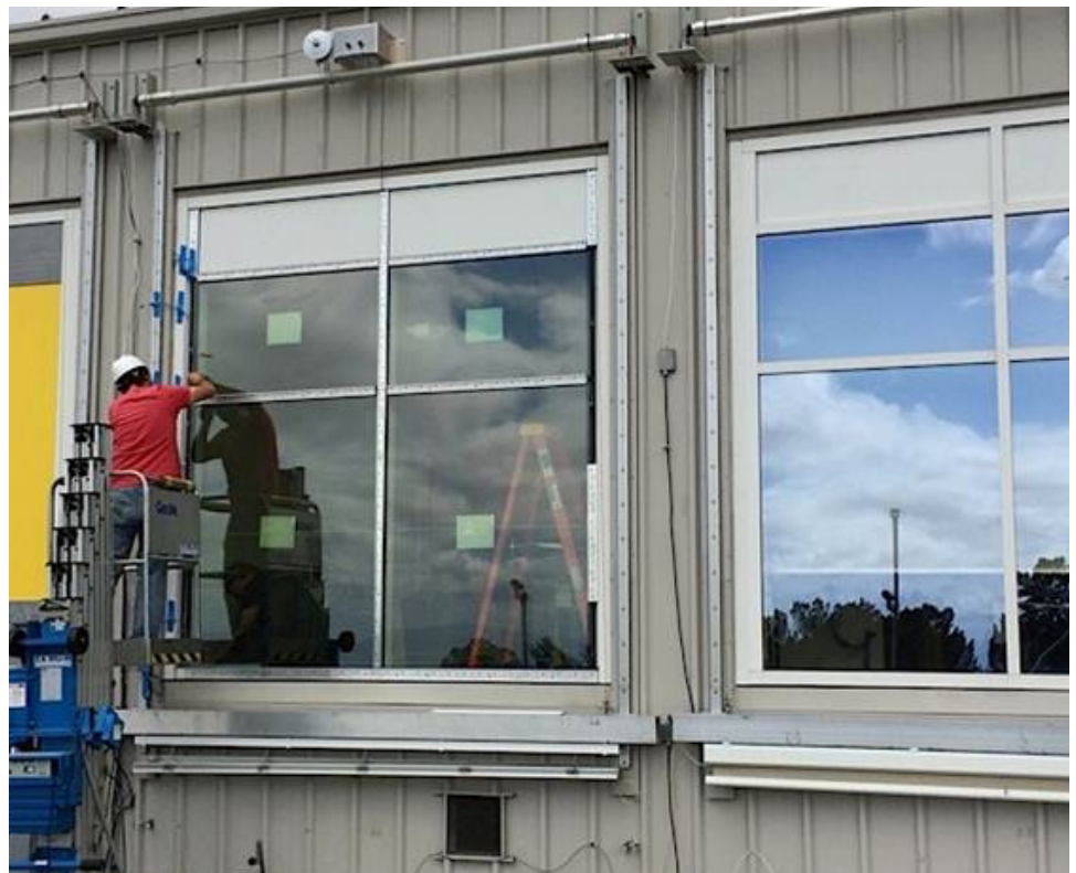
Installing energy-efficient windows Photo Credit: U.S. Department of Energy
