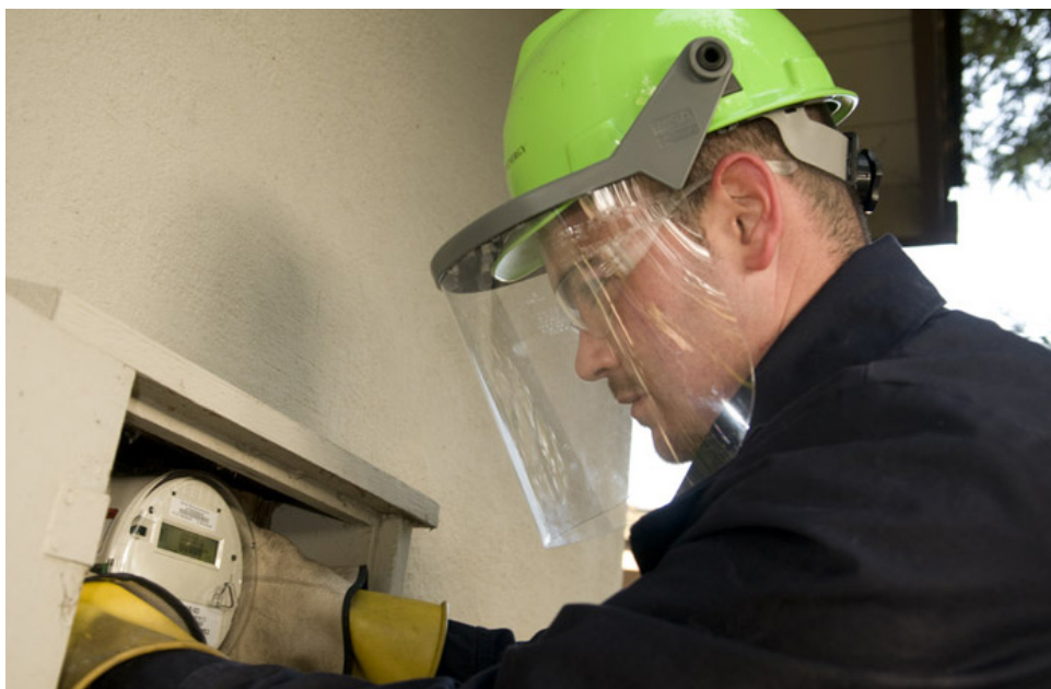
Installing a residential smart meter Photo Credit. pgegreenenergy / Foter / CC BY
