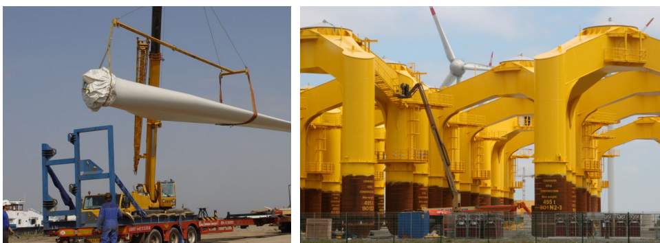
(Left) Transporting a wind turbine blade, Photo Credit. Evert Kuiken / Foter / CC BY-ND (Right) Tripile offshore wind turbine foundations, Photo Credit. U.S. Department of Energy
