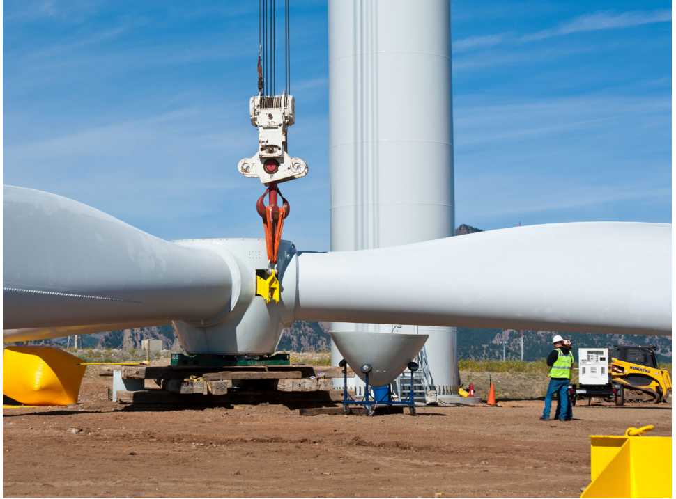
Drawing a wind turbine up for placement Photo Credit. Dennis Schroeder / NREL
