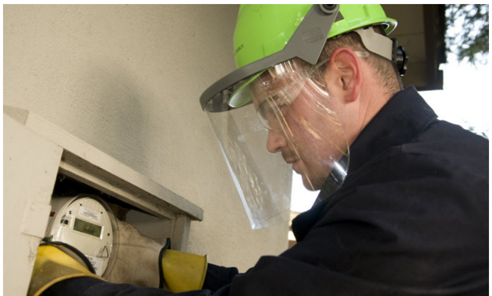
Installing a Smart Meter
